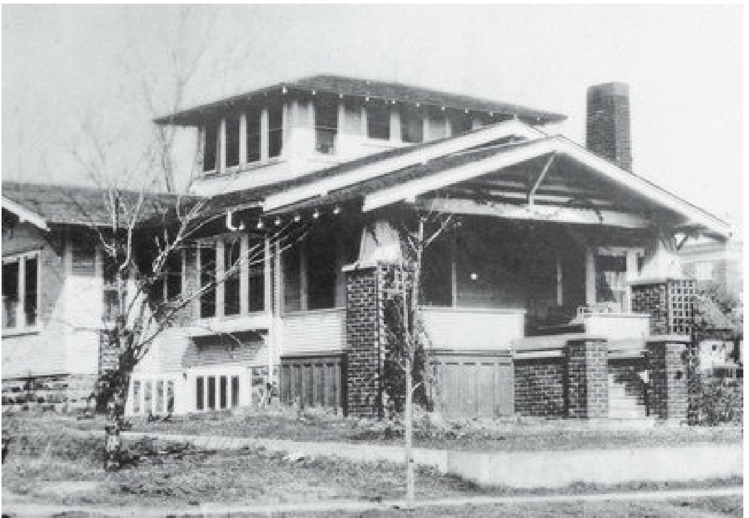
.... Rita and Bill Smith's house before the blast—and then after Credit 30
