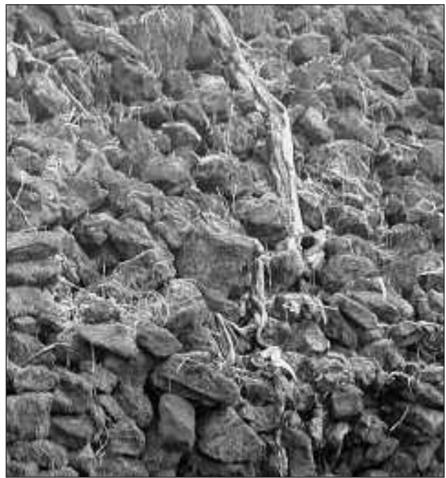
Figure 5. The foundation structure and original wall of first platform on the South side (Photo Paul Wallin)
