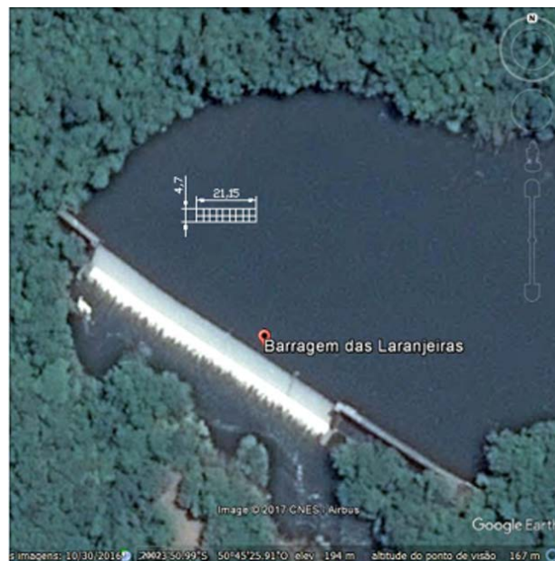
Figure 2. Image of the Laranjeiras Dam.
