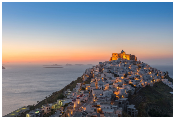
Figure 7. A view of the main settlement of Astypalea, known as Chora [24].
