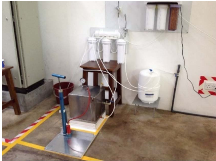
Figure 2. Air operated domestic use brackish water reverse osmosis plant.
