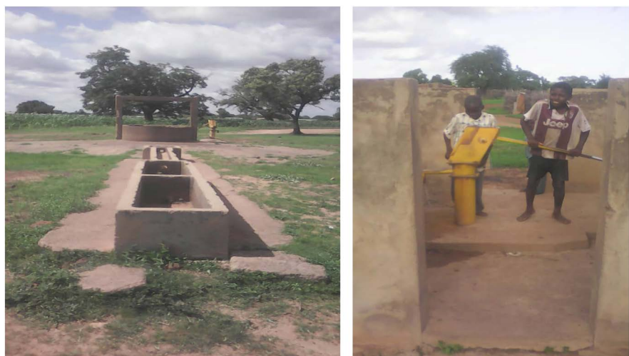
Photo 4. Large-diameter well and human-powered pump in the Municipality of Fagui and Tempéla.
