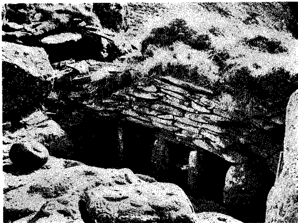
1. HOUSES NOS. 40 TO 43.
