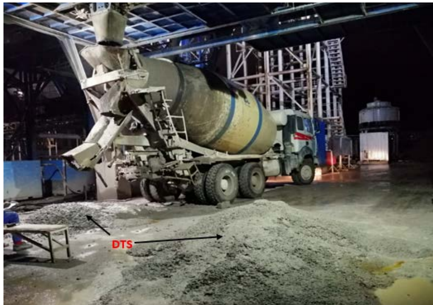
Photo 3. Discarded test samples (DTS) from concrete batches.
