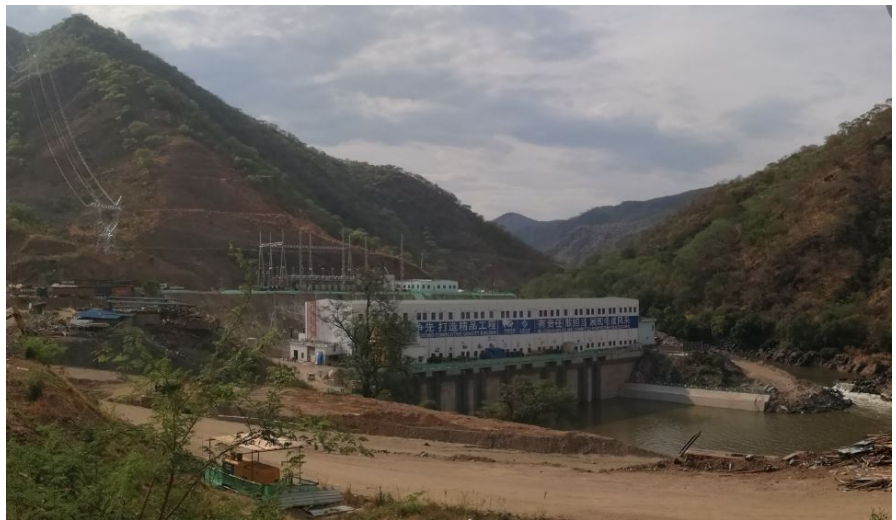
Photo 12. Powerhouse and 330 KV Switch yard (tailrace view).
