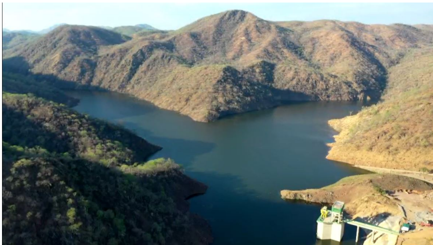
Photo 9. KGL Dam (intake view with water filled dam).
