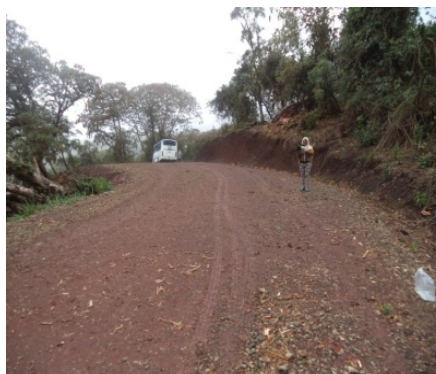
Figure 5. Partial view of road construction.
