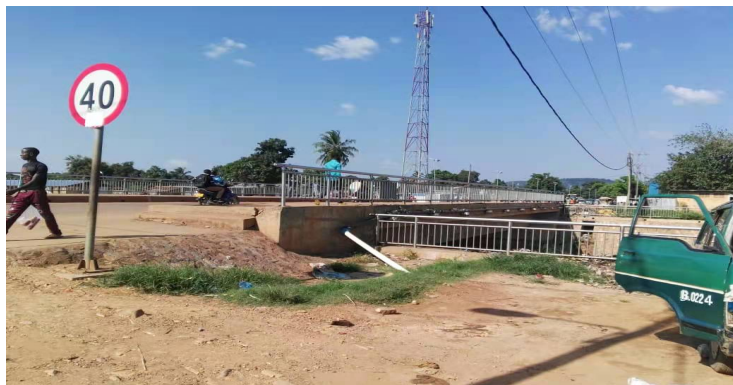
Photo 7. Sapeke Bridge. Source: Central African Republic government official site.
