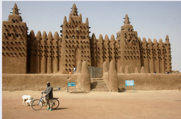
Figure 9.9 | The Great Mosque in Djenne | The Great Mosque in Djenne demonstrates the regional architectural style of the Western Sudan. The original structure was likely built in the thirteenth century. The current mosque was rebuilt in the early twentieth century. The wooden scaffolding gives the structure support and also helps men replaster the exterior, which they do every year. The exterior of the mosque is plastered in mud (adobe).
